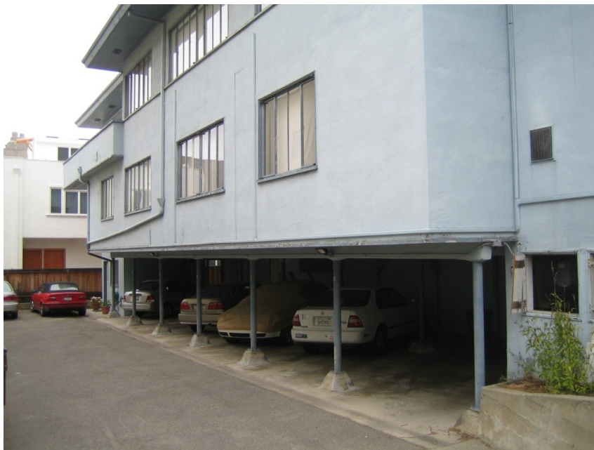
Figure 1. Photo of an example soft-story property in Berkeley. Photo credit: Sharyl Rabinovici, May 2010.
